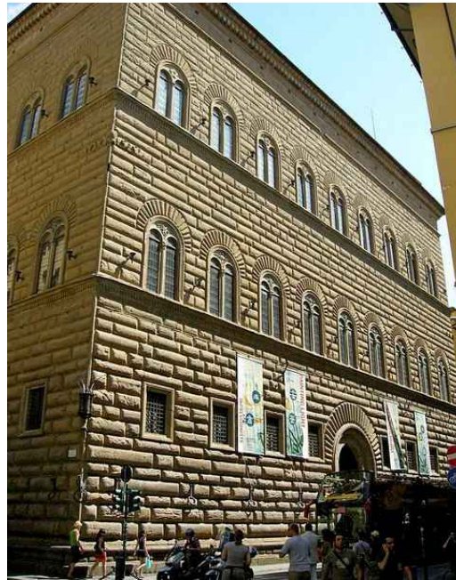
Street facades of the Palazzo Strozzi in Florence, Italy (1489-1504)
