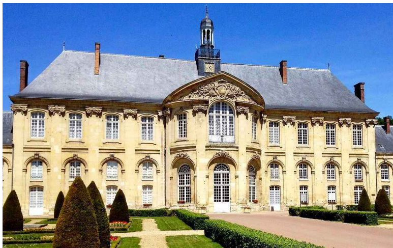
Main building of Prémontré Abbey, near Laon, Aisne, France (1718) - unknown architect
