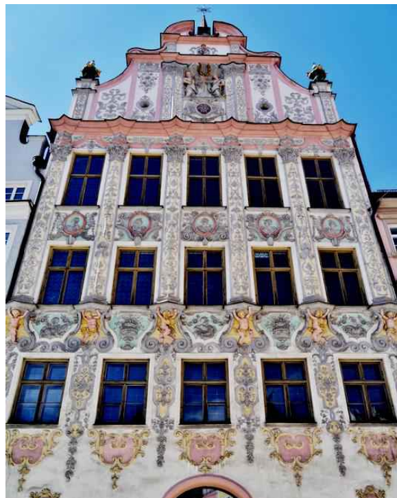
Dominikus Zimmermann: facade of the Landsberg am Lech town hall (Bavaria, Germany), 1719
