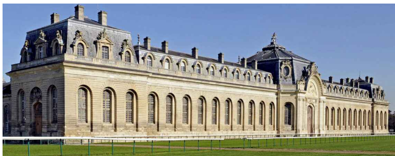
Jean Aubert (known as Aubert aîné): Grandes Écuries building at château de Chantilly, France (1719-1735)
