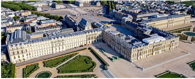
Jules Hardouin-Mansart: modifications to the garden facade and side extensions of the Château de Versailles (1678-1689)
